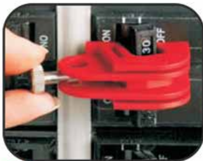
1 Tighten set screw
