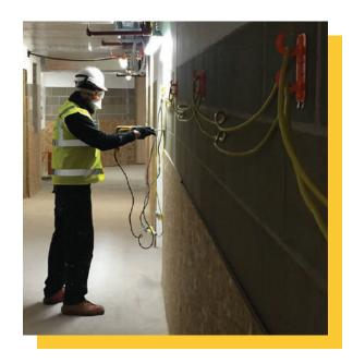
The new wiring regs come into effect in January 1, 2019. The 18th Edition states that plastic fixings cannot be used as the sole use of holding up cables. However, the IET states:
